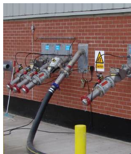
Pneumag installed at bulk material intake, ATEX rated.
