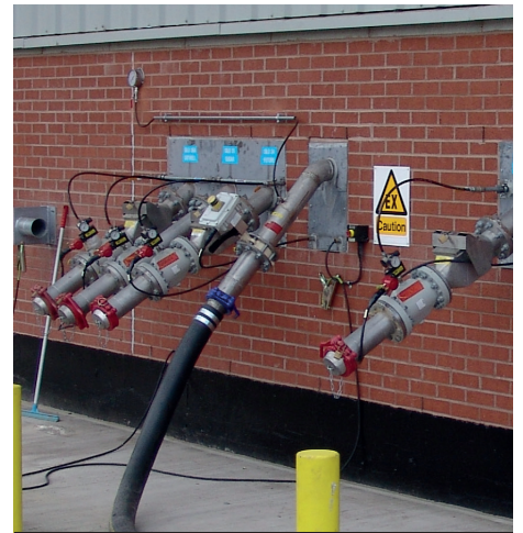
Pneumag installed at bulk material intake, ATEX rated.
